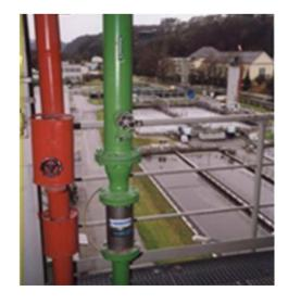
Since 1997, Wacker-Chemie's engineers had installed numerous ScaleBuster® conditioners right before the heat exchangers or downstream from the pumps to protect the heat exchangers, pumps and other pieces of equipment in the processes.
